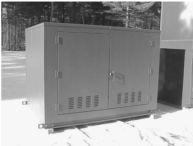
FIGURE 6.3 Example padmounted capacitor. (From Northeast Power Systems, Inc. With permission.)
