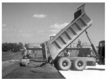
A flat-bed dump truck delivers concrete directly to the pavement bed
