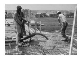
Conveying concrete by pumping
