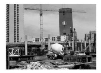
Using a tower crane and a bucket for conveying concrete
