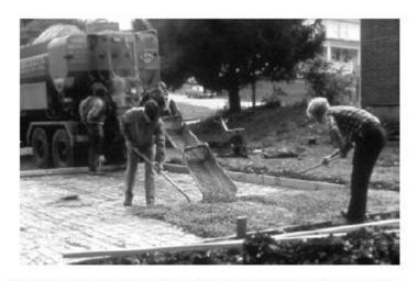
Use of a mobile concrete batching and mixing truck to produce concrete at the job site
