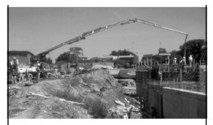
Use of boom and pump to place concrete to a wall
