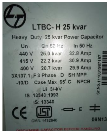
Figure 6.3 Typical name-plate of power factor correction capacitor
